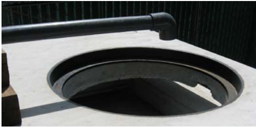
Figure 3 Influent to TreePod® Filter via the Manhole Access
